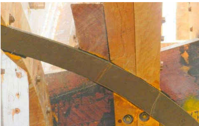
Metal diagonal strap attached after keel.
