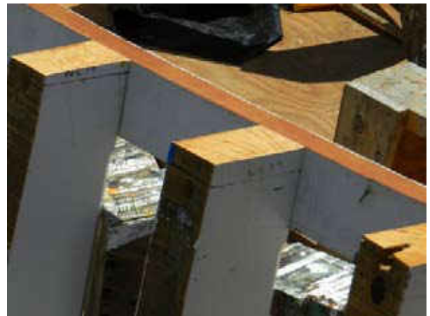
Main deck stanchions ready for planking and rails.
