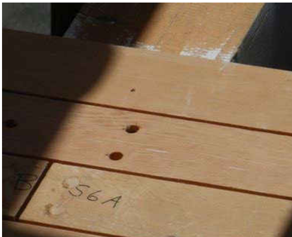
Main decking is started.
